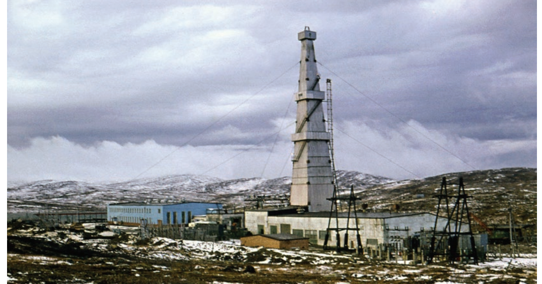
Gigantic drill housing built by the Soviets for their Kola project.
