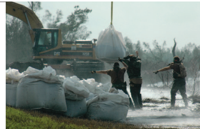
Army engineers repair a break in the levees.
